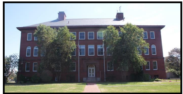
Town Hall Renovations, 2010
